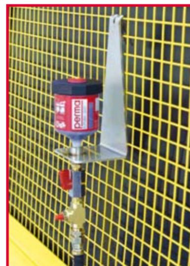
CH01 bracket with 708V manual purge kit
